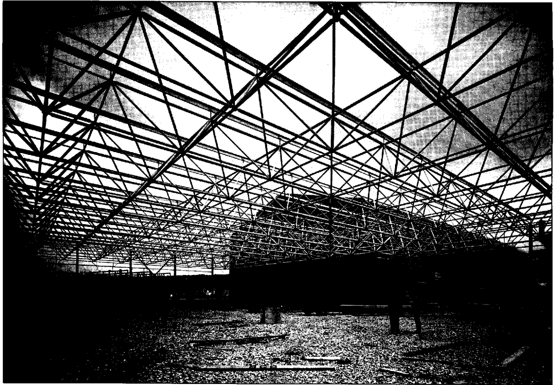
Fig. 3.37 A Mero space frame, supported around its perimeter, acts as the roof structure in this single-storey building. Note the vertical-plane diagonal bracing elements which must be provided in each external wall of the building. The fully triangulated space framework acts as horizontal-plane bracing. [Photo: BICC]
