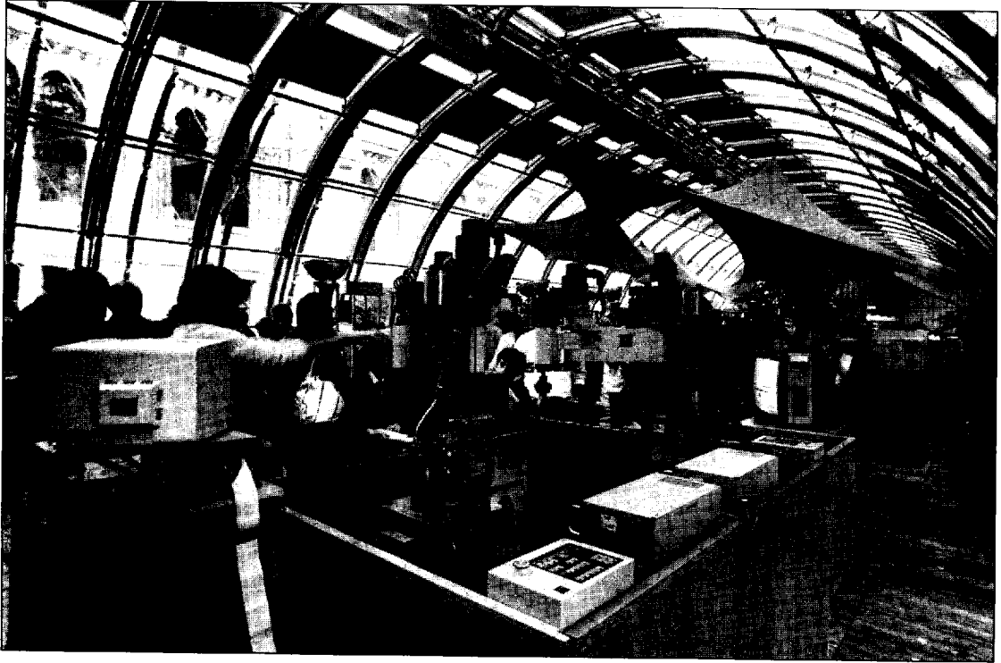
Fig. 1.12 Building for IBM Europe travelling exhibition. Renzo Piano, architect/engineer. Ove Arup and Partners, structural engineers. A complex, highly efficient vaulted structure like this would not normally be used for a short-span enclosure. It was justified in this case due to a requirement for a lightweight structure for a portable building. The choice of lightweight materials – timber and plastic – was also sensible. [Photo: Ove Arup & Partners]
