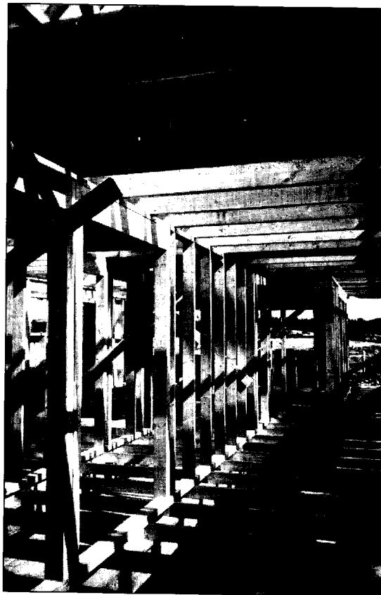
Fig. 1.19 Timber loadbearing-wall structure. Everything here is structural. The wall and floor structures consist of closely spaced timber elements. Temporary bracing elements, which provide stability until non-loadbearing cross-walls are inserted, are also visible. [Photo: A. Macdonald]
