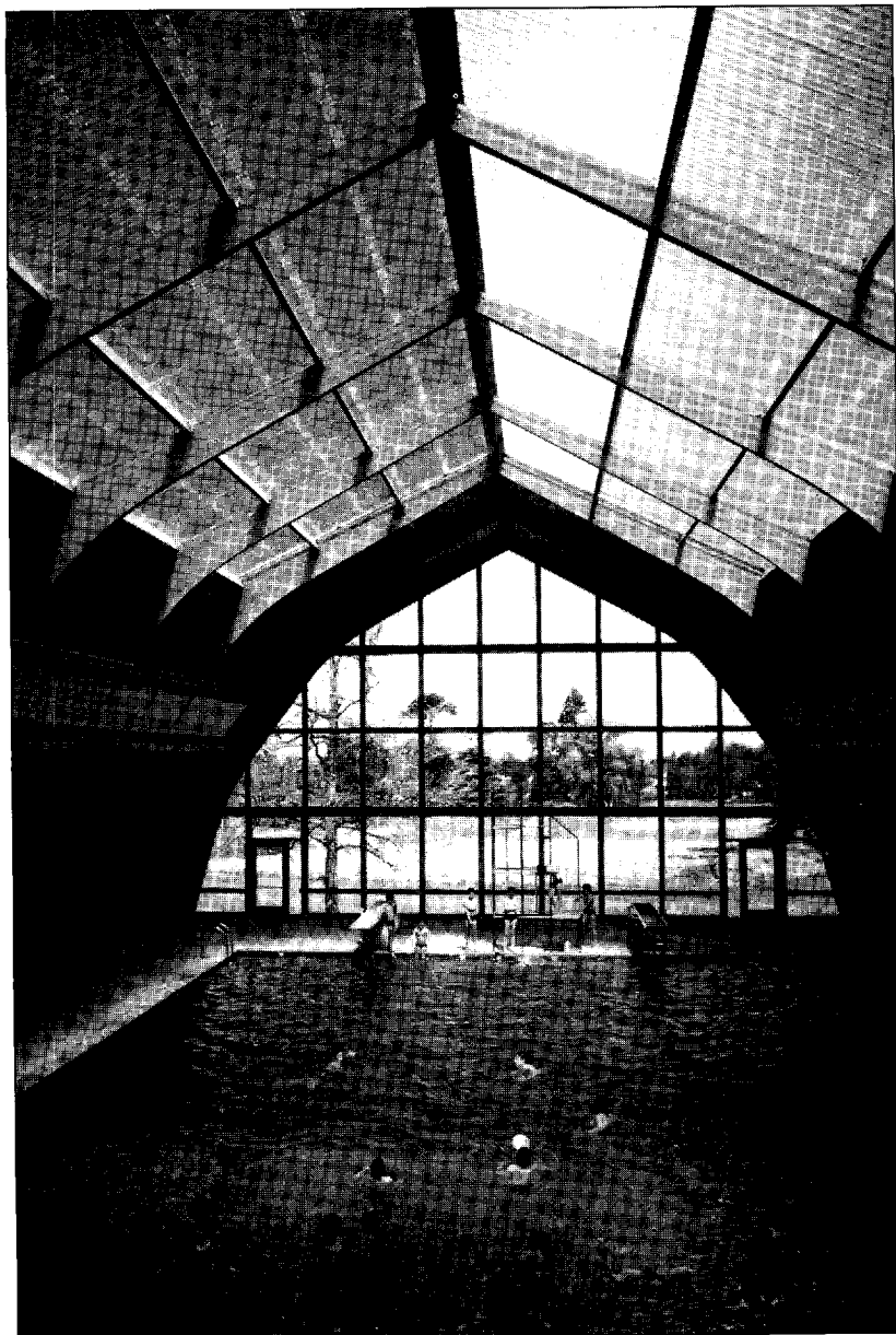
Fig. 6.3 Primary–secondary system. The primary elements here are laminated timber portal frames. These carry purlins which in turn support the roof and wall cladding.
