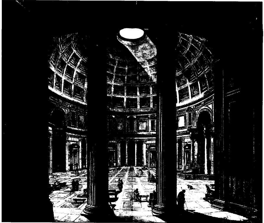
Fig. 5.11 The Pantheon, Rome, 2nd century CE. This was the largest domed structure of Roman antiquity. The coffering of the inner face of the dome and voiding of the walls suggest that the 'architects'/engineers' responsible for this building had a good intuitive or empirical understanding of the structural behaviour involved. They used these features to excellent architectural effect. [Copyright: RIBA Photo Library]
