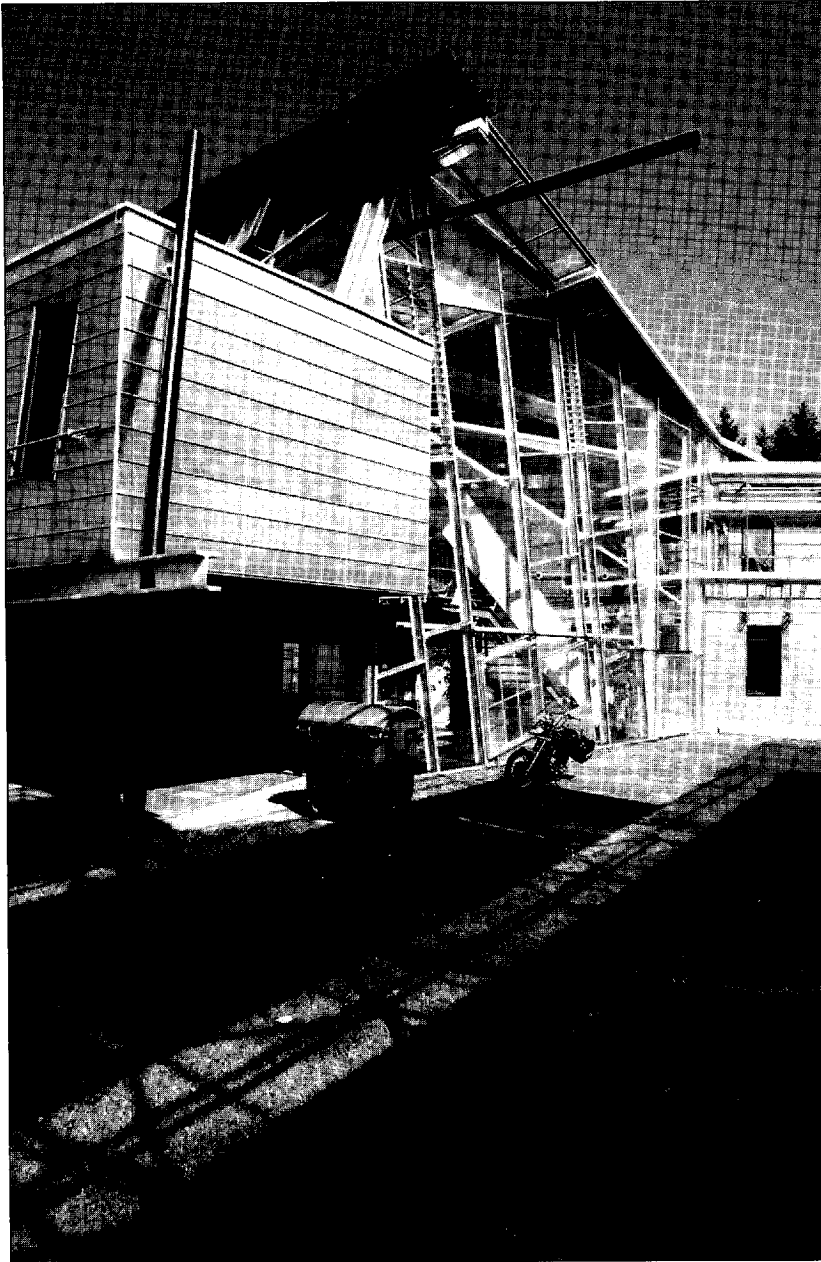
Fig. 2.2 Solar Research Institute (Hysolar), Stuttgart, Germany, 1988–89. Gunther Behnisch & Partner, architects. The irregular geometry and large areas of glazing required that a skeleton framework structure be adopted to support this building. The choice of steel produced a particular aesthetic quality – the most notable aspects of this are the slenderness of the structural elements and the refined appearance of the exposed steelwork. [Photo: E. & F. McLachlan]
