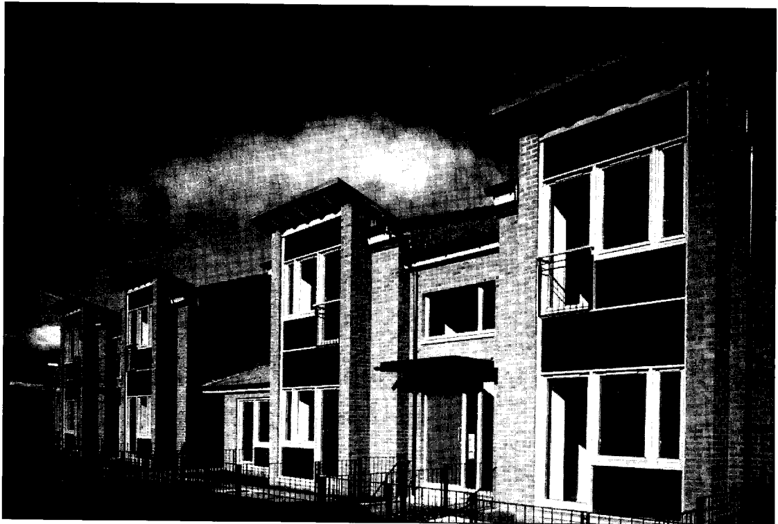
Fig. 1.10 Housing, Gogarloch Syke, Edinburgh, Scotland, 1996. E. & F. McLachlan, architects. These houses are good examples of panel structures in loadbearing masonry. [Photo: Keith Hunter, copyright: E. & F. McLachlan]
