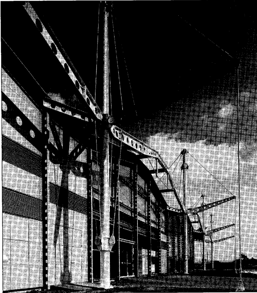
Fig. 2.6 Renault Warehouse and Distribution Centre, Swindon, England, 1983. Foster Associates, architects, Ove Arup & Partners, structural engineers. Many of the features which are associated with high structural efficiency are visible here, such as the semi-trussing of the main elements, the use of tapered profiles, the I-shaped cross-sections and the circular lightening holes. They were adopted for visual reasons, however, as few of these complexities can be justified on technical grounds due the relatively short span involved. [Photo: Alastair Hunter]
