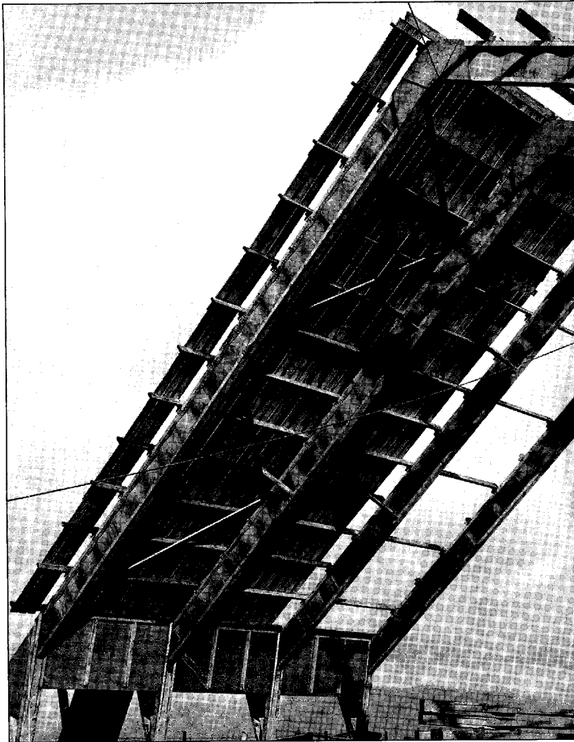
Fig. 6.53 Single-storey timber skeleton-frame structure in which the principal elements are plyweb built-up-beam sections.
