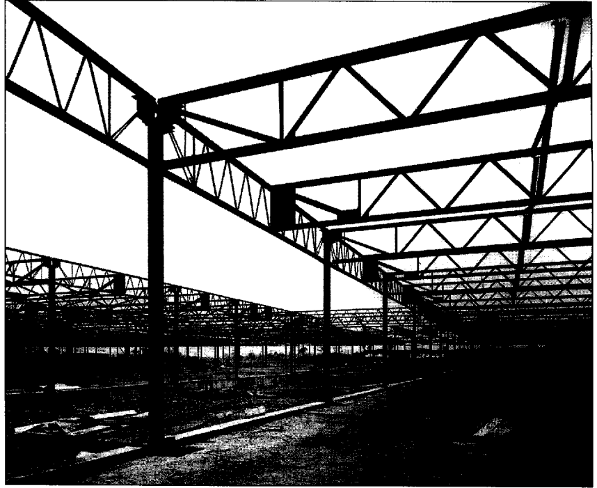
Fig. 3.26 A single-storey steel framework is shown here comprising lightweight Metsec joists based on cold-formed sections. [Photo: Photo-Mayo Ltd]
