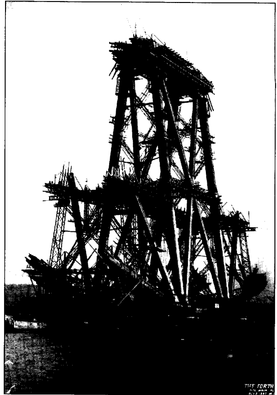
Fig. 1.21 Forth Railway Bridge, Scotland, 1882–90, Henry Fowler and Benjamin Baker, engineers. The main part of the structure consists of three pairs of balanced cantilevers. In this shot the central tower of one pair of cantilevers has been completed and the first elements of the cantilevers themselves have been added. The arrangement was adopted so that the uncompleted structure could be self-supporting throughout the entire period of construction. [Photo: E. Carey; copyright: British Rail Board Record Office]
