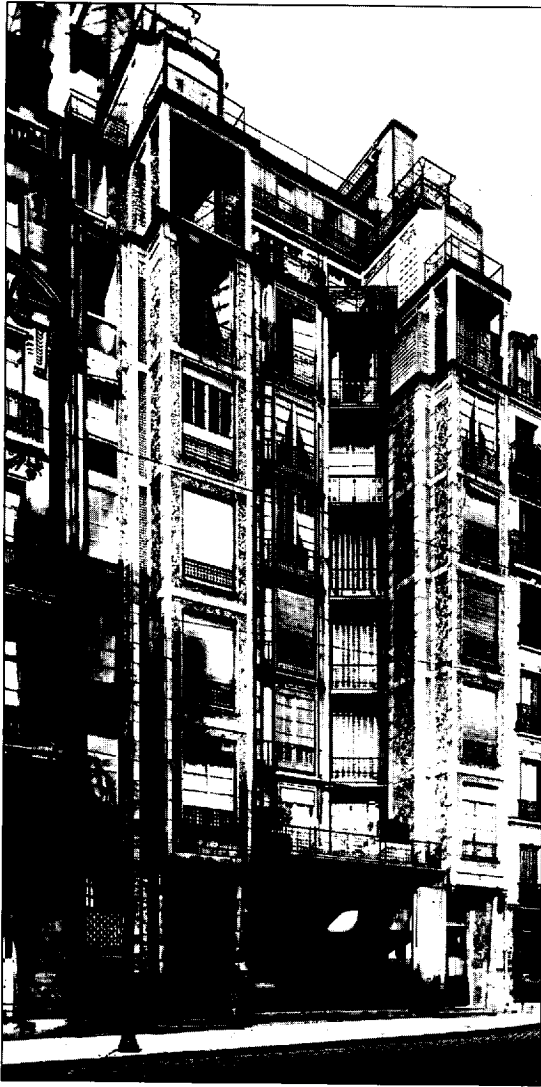
Fig. 4.4 Apartment block, 25 bis rue Franklin, Paris, 1902–05, Auguste Perret, architect. By using a reinforced concrete frame structure Perret was able, with this building, to redefine the layout and fenestration of the traditional Paris apartment. The building also made a significant contribution to the development of a new architectural aesthetic based on the technology of the skeleton frame.
