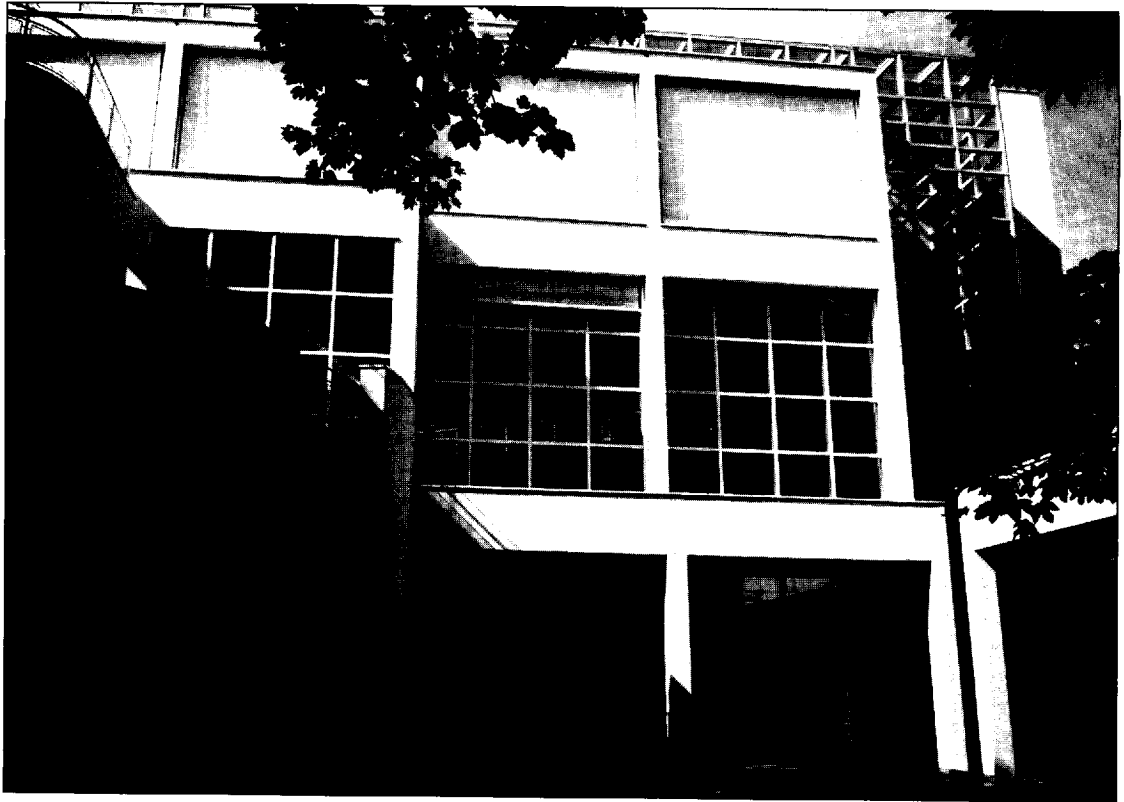
Fig. 4.18 Museum of Decorative Arts, Frankfurt on Main, Germany, 1979–85. Richard Meier, architect. The juxtaposition of solid and void and of rectilinear and curvilinear elements is typical of the work of Richard Meier. In situ reinforced concrete is an ideal structural material for this type of architecture [Photo: E. & F. McLachlan]
