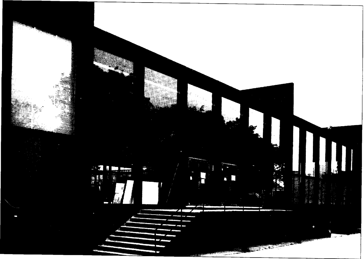
Fig. 1.2 Crown Hall, IIT, Chicago, USA, 1952–56. Ludwig Mies van der Rohe, architect. This building has a steel-frame structure. The glass walls are entirely non-structural.
