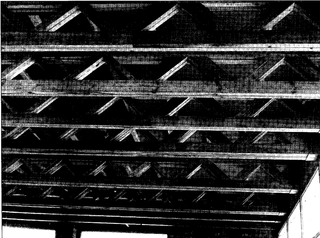
Fig. 6.26 Built-up lattice beams. Proprietary components such as these are used, like plyweb beams, to extend the span ranges of traditional forms of timber construction.
