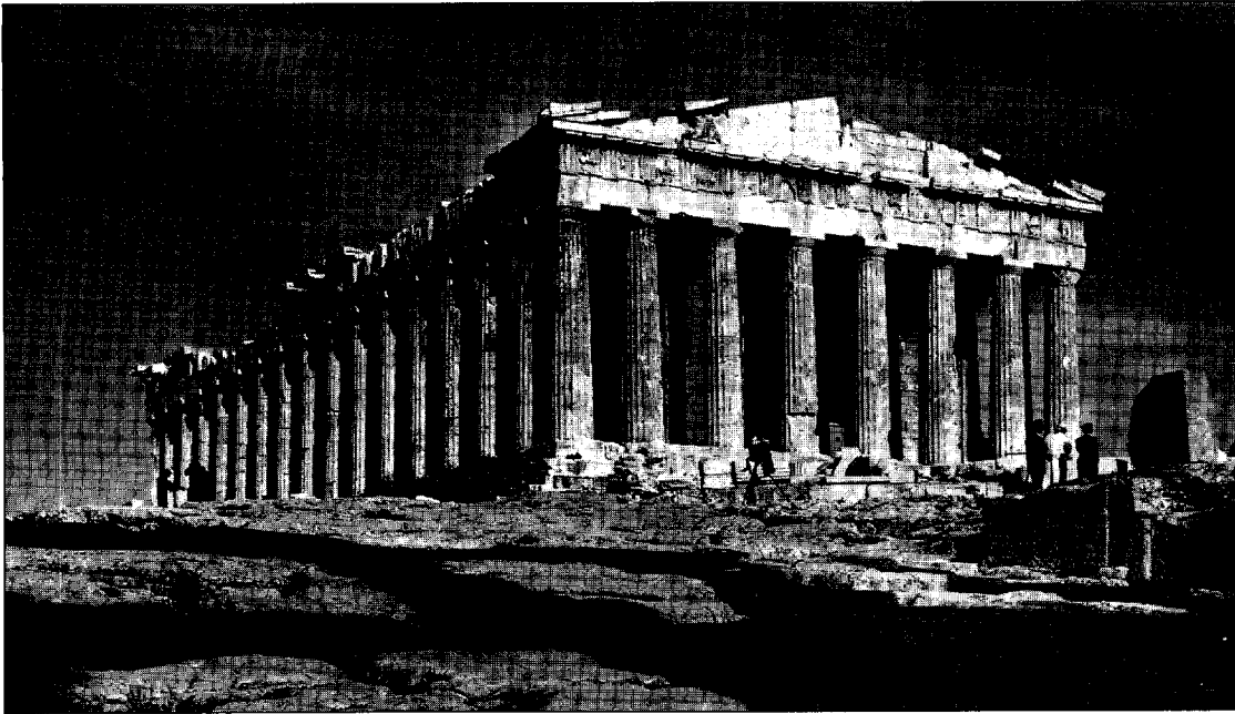
Fig. 5.15 The Parthenon, Athens, 5th Century BCE. This is the most refined example of post-and-beam construction in the Western architectural tradition. The short spans involved are a consequence of the inherent weakness of masonry in tension and therefore in bending. [Copyright: RIBA Photo Library]
