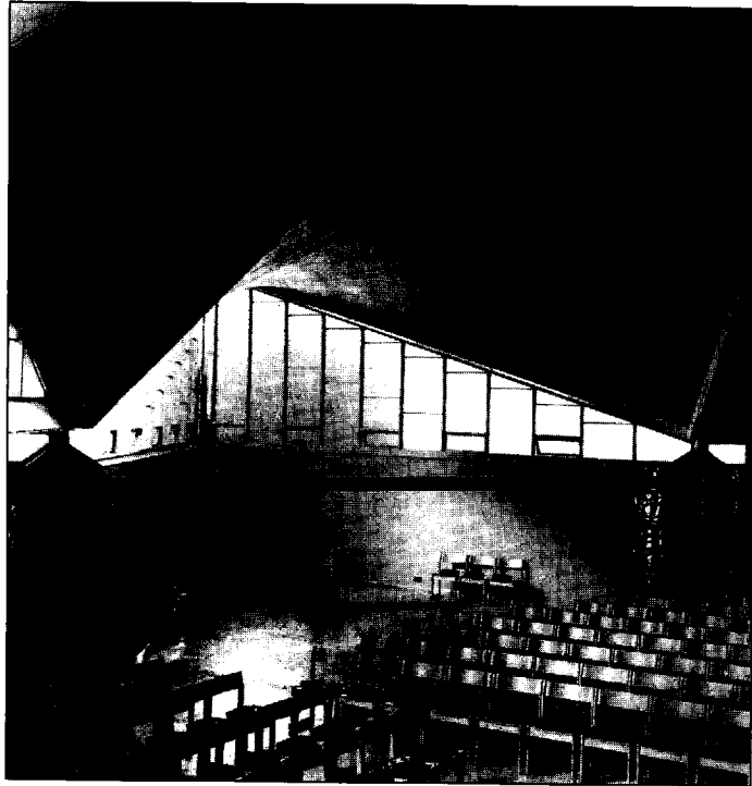
Fig. 6.59 Timber hyperbolic paraboloid shells are used here to form a roof structure of distinctive shape.
