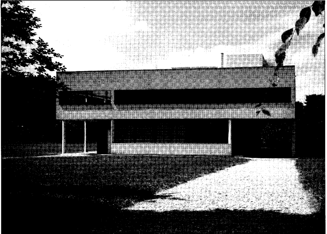
Fig. 4.6 Villa Savoye, Poissy, France, 1929. Le Corbusier, architect. The technology of the reinforced concrete framework contributed significantly to the visual language developed by Le Corbusier in the 1920s. [Photo: Andrew Gilmour]
