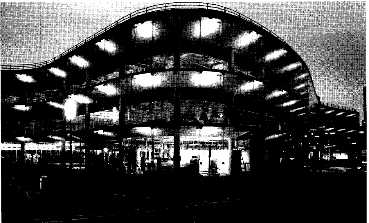
Fig. 4.17 Willis, Faber and Dumas office, Ipswich, England 1974. Foster Associates, architects, Anthony Hunt, structural engineer. The curvilinear plan, cantilevered floor slabs and transparent walls of this building give architectural expression to the structural properties of reinforced concrete (Photo: Alastair Hunter).
