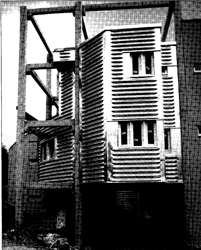
Fig. 1.8 Nenfildweg Housing, Graz, Austria, 1984–88. Gunther Domenig, architect. The structure of this building is a reinforced concrete framework. Its adoption has allowed greater freedom to be exercised in the internal planning and external treatment than would have been possible with a loadbearing-wall structure. [Photo: E. & F. McLachlan]
