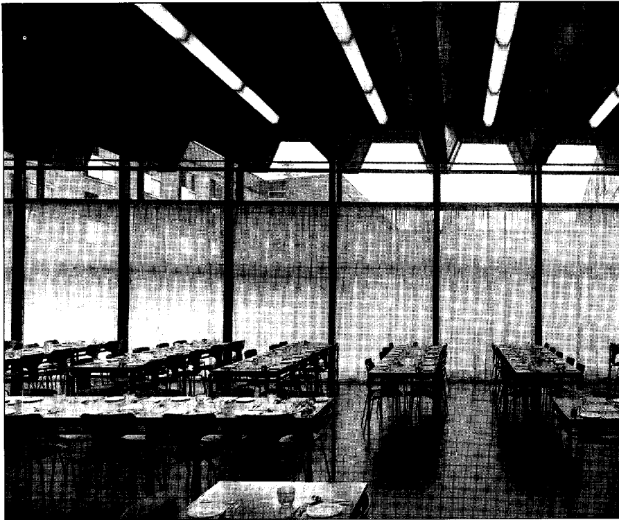
Fig. 6.58 Timber folded-plate structure. Forms such as this, which are constructed from panels consisting of two skins of plywood separated by sawn-timber stringers, have good structural properties and allow long spans to be achieved.
