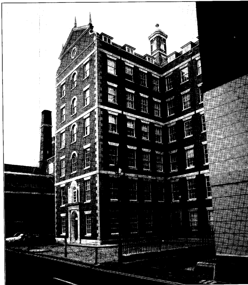
Fig. 1.1 Offices, Dufour's Place, London, England, 1984. Erith and Terry, architects. As well as having a space-enclosing function the external walls of this building are the loadbearing elements which carry the weights of the floors and roof. [Photo: E. & F. McLachlan]
